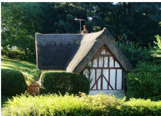
Picture 4. Unusual 17th century single storey thatched property with later fake timbering applied.
